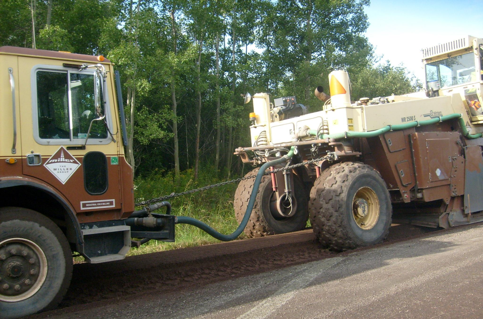
Stabilizing Pulverized Base
